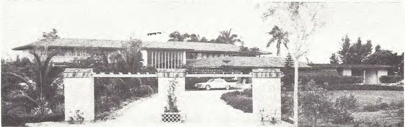
Seen at a distance, the most remarkable feature of the Groves home is the green tile roof that blends with natural colouring of surrounding sea, sky and landscaping.
